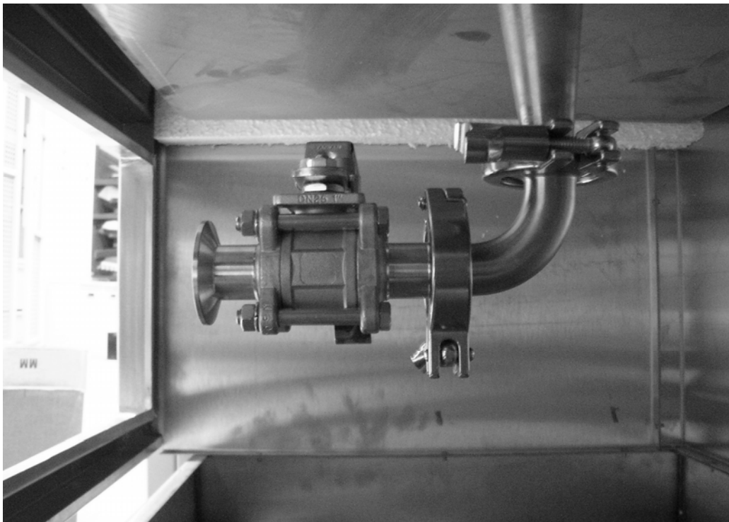
Optional Stainless Steel Ball Valve Kit DC-SVK Installed
