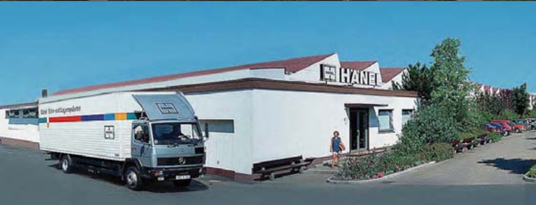
Hanel plant 1 Bad Friedrichshall, Germany
